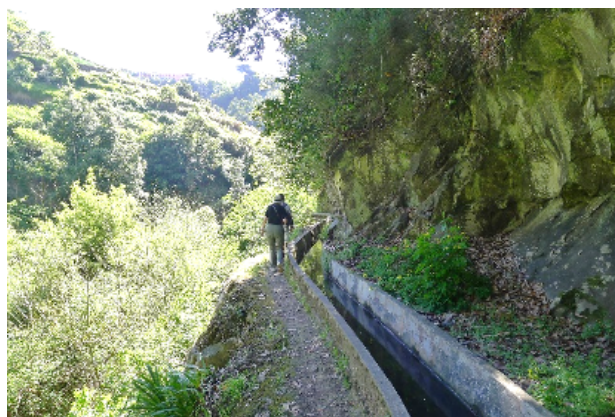
Walking a typical levada (water channel) in the hills above Funchal; they bring water condensed from clouds in the high mountains above down to the dry southern coastal areas.
