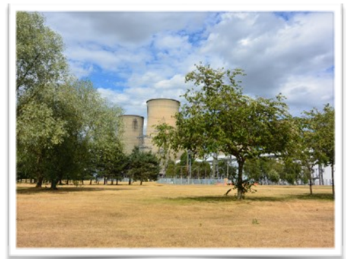
Eggborough Power Station, North Yorkshire
